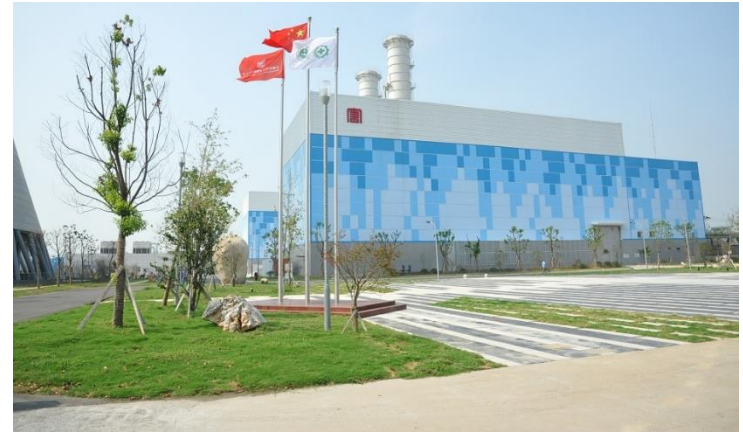
Gas-fired Power Plants
