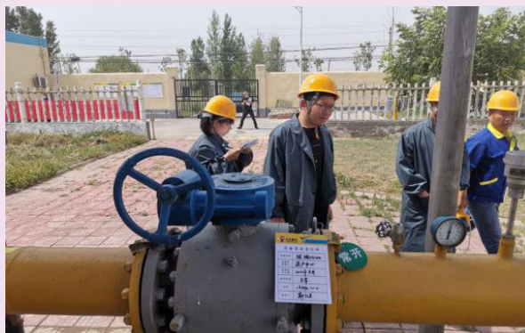
A scene of the joint safety inspection of Hebi Company.
