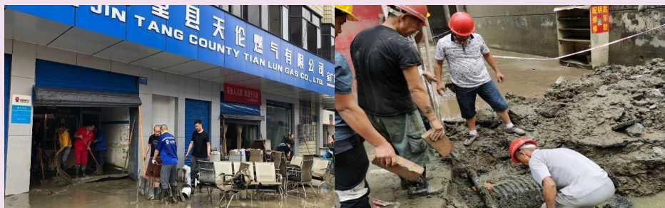
Jintang Company participated in rescue and relief work on the site.
