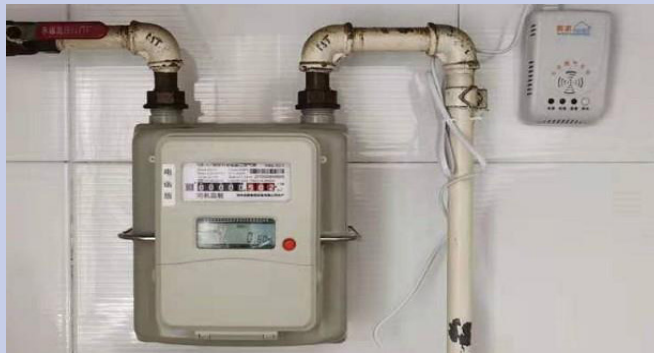
A meter-alarm integrated device developed jointly by the Group and Chuangyuan Company.
