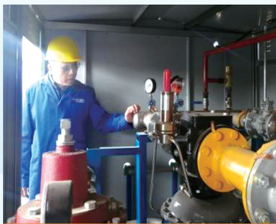
Safety inspection of Tian Lun Gas
