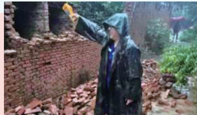
Hebi Company inspects gas leakage on the collapsed site
